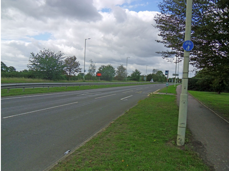
Goldington Road between the two roundabouts looking west
