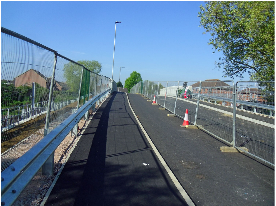
Footpath and carriageway in late April looking westwards leading up to the bridge
