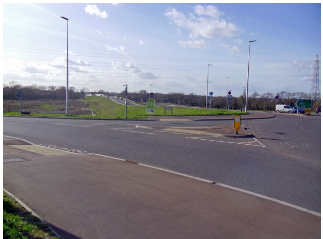
Existing dangerous crossing
