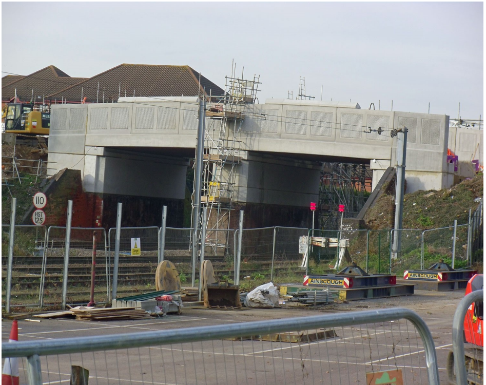
Upgraded bridge as of November 2019
