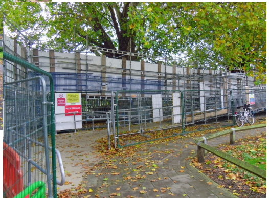
Temporary bridge - stepped access in Spencer Road for able pedestrians
