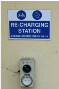
Charging point at The New Inn Shalfleet IoW
