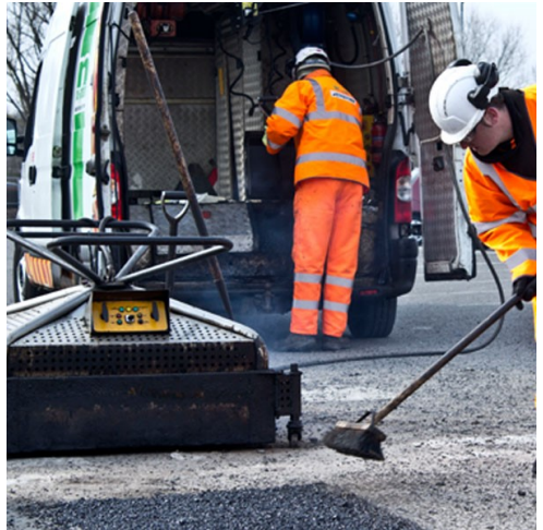
Thermopatcher in action
