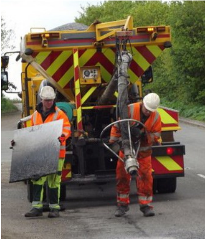
Thermopatcher in action
