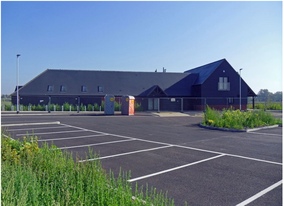
General view of the pavillion with the cycle stands to the left
