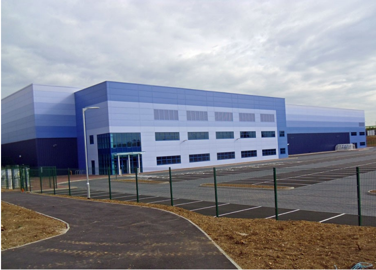
View of the building from the west showing the stands and the cycle/ pedestrian route from Cambridge Road to the entrance.
