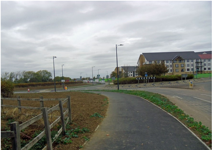
New cycle track around west arm (left) of roundabout with new retirement village on far right
