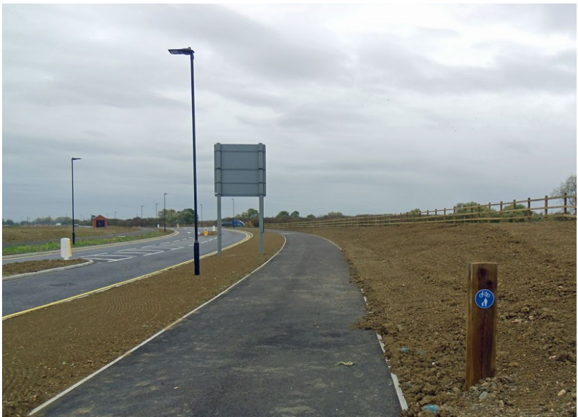
New road, from roundabout to Logistics Park, still to be opened, with 3.5 metre cycle tracks on each side separated from carriageway by generous verges
