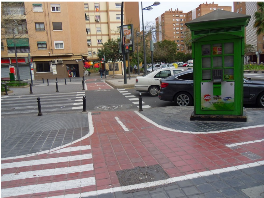
Typical two way off-road cycle track with parallel crossing of main road
