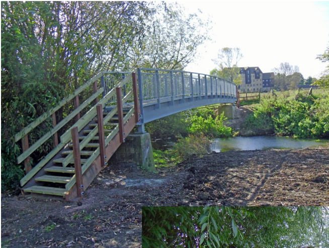
New metal bridge
