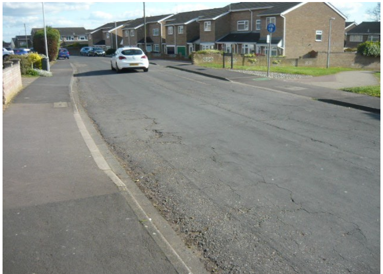
Original unmarked crossing
