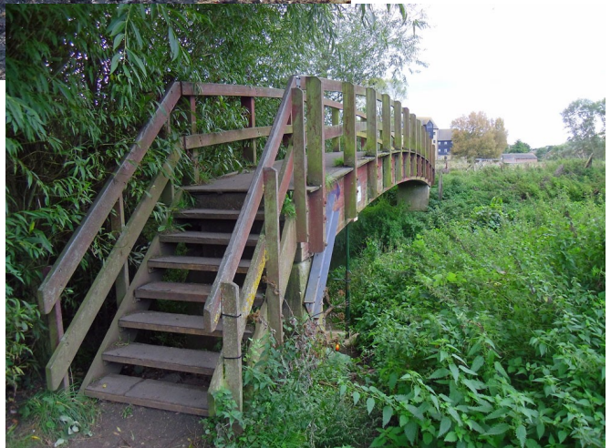
Old bridge with strengthening plate on side and held up by two metal props
