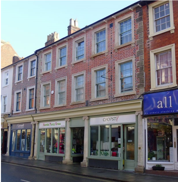
99-101 High Street built ~1860s with central alley to Howard Street
