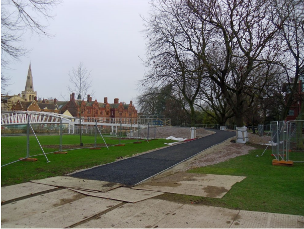
On the south side (left) in St Mary's Gardens the two ramps leading to the new bridge are currently being done
