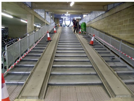
Stairs/wheeling channels to upper floors
