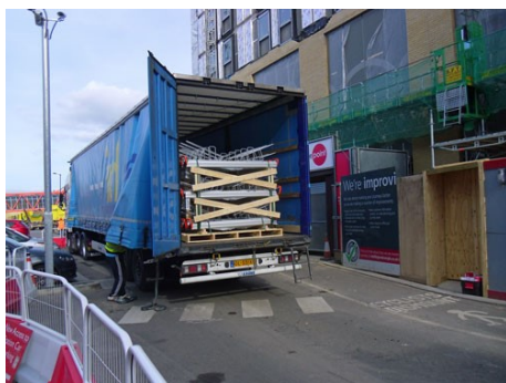
Further racks arriving from the Netherlands
