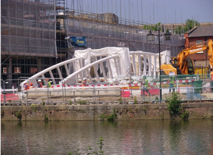
Bridge being assembled
