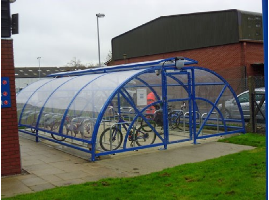
40 space cycle shelter next to King's Place Office Block
