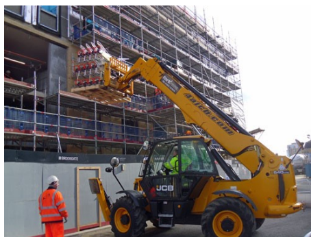
Racks being lifted to second floor
