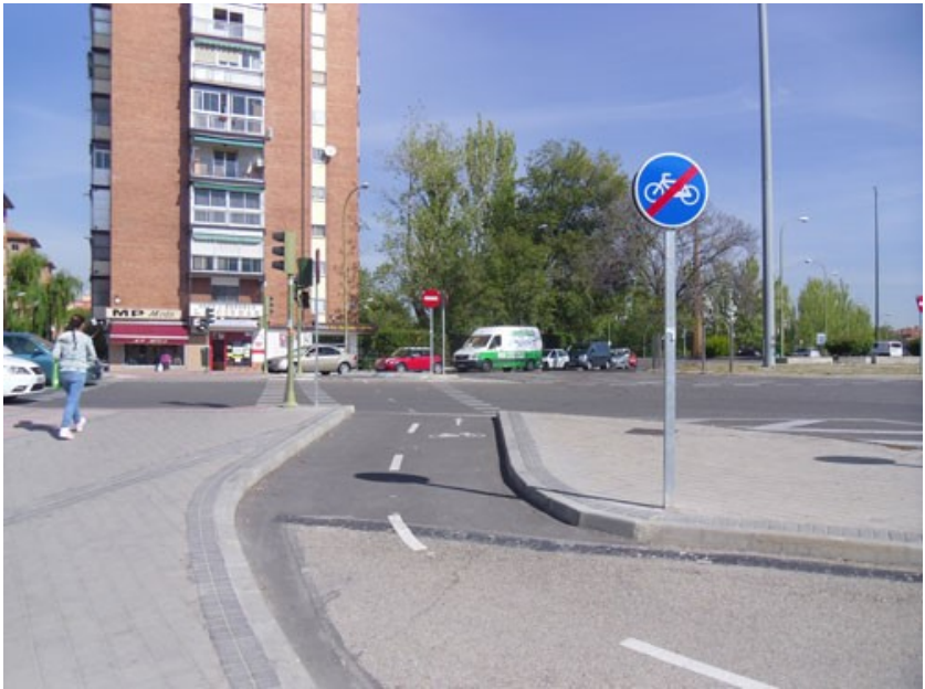
Two way off-road cycle track crossing busy road at signals
