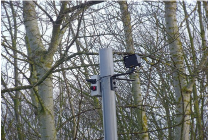
Sensor on a separate pole at the south east end of the bridge. The one on the north side is attached to the traffic signal pole outside the Anchor Inn
