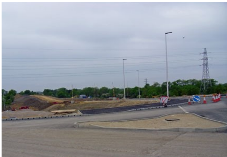
Cycle track under construction at Clapham Road end of link
