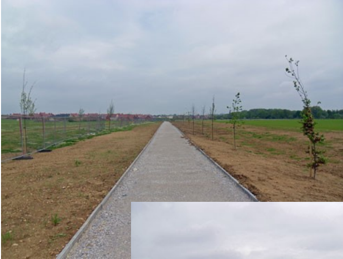
New cycle track under construction disappearing into the distance
