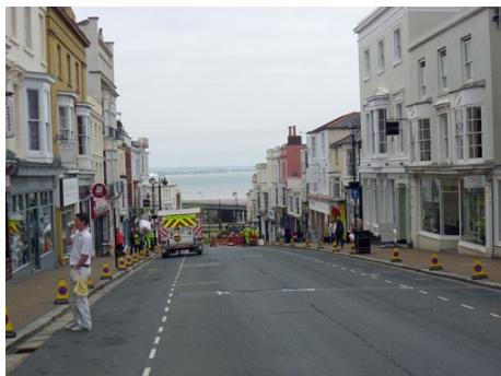
Union Street being repaired
