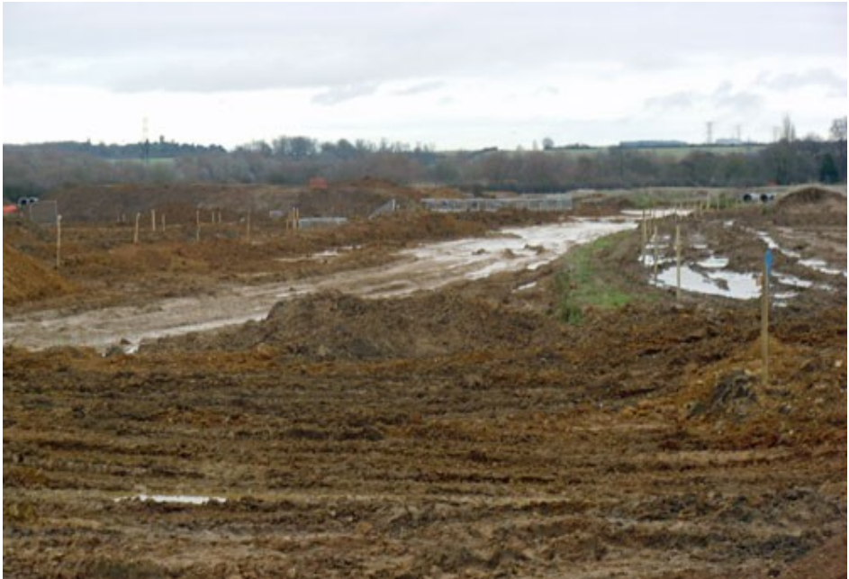
General muddy conditions under which contractors have to work
