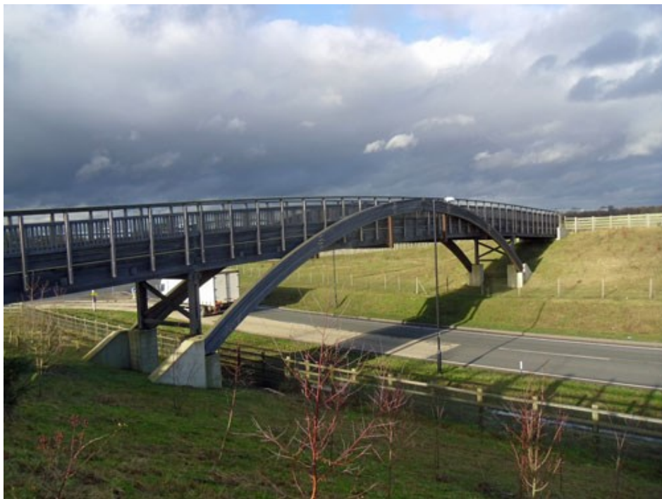
Wooden Bridge carrying a bridleway across Ridgmont Bypass
