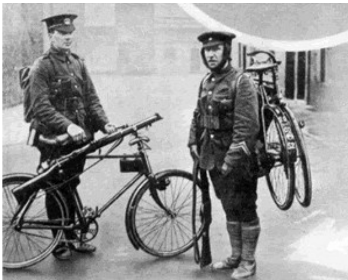
Men of the Lancashire Fusiliers (Cyclist Corps) with BSA folding bicycles which can be folded and hung on their backs in one and a half minutes
