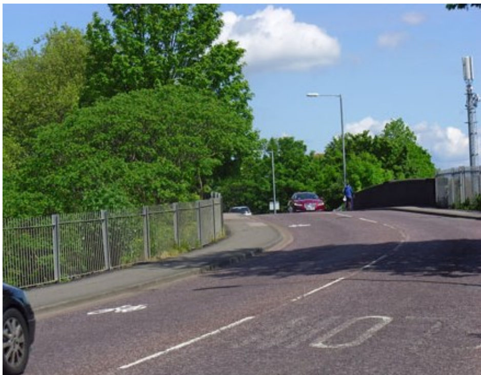
Bromham Road railway bridge approach going east
