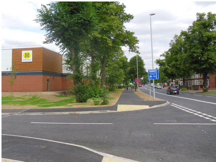
View of dual use track and bus lane looking north from uncontrolled delivery road
