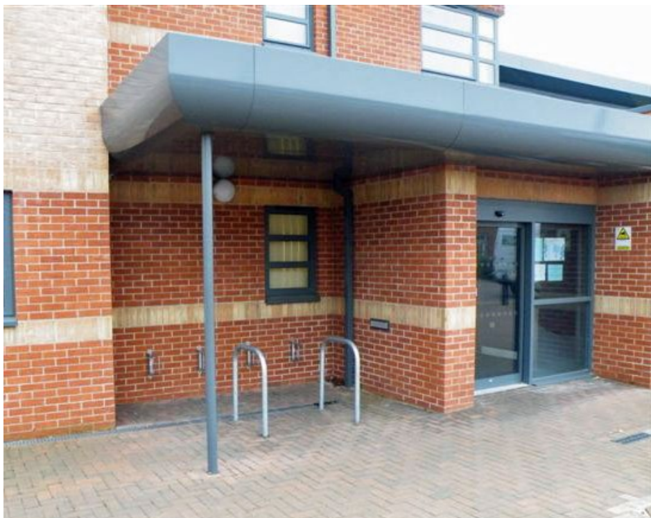
The Glebe Surgery Clapham Two 'Sheffield' stands replacing the original four 'Butterfly' stands
