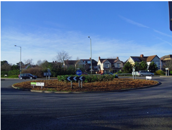
Newnham Avenue/ Barkers Lane roundabout from Barkers Lane side central reservation
