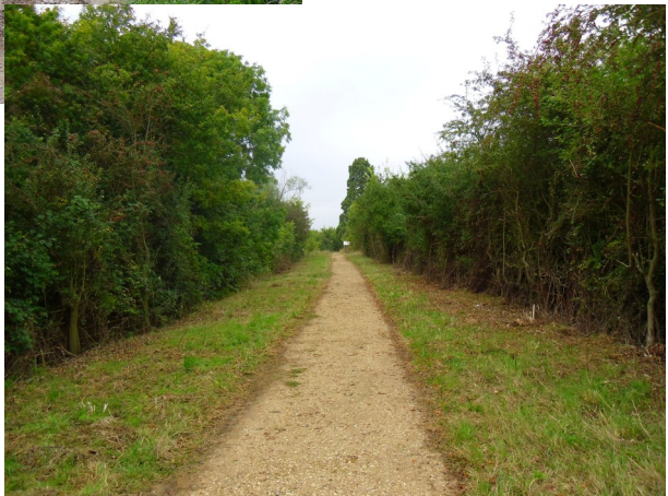
track after repair and hedge trimmed and vegetation cleared
